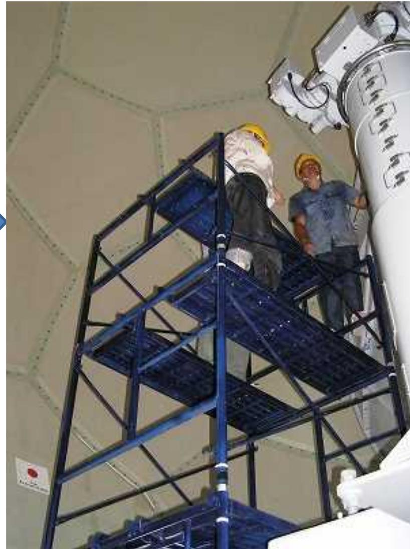
Replenish grease, replace oil, check belt tension and function switch of antenna
