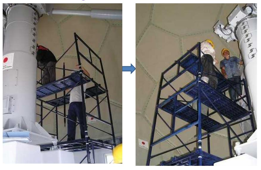
Replenish grease, replace oil, check belt tension and function switch of antenna
